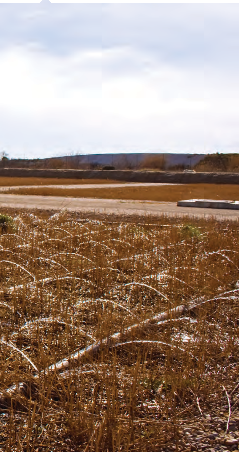
Constructed wetlands for wastewater treatment plant
