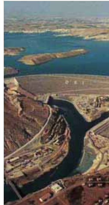
The Atatürk Dam (Turkey) is the largest in a series of 22 dams and 19 hydroelectric stations built on the Euphrates and Tigris rivers
