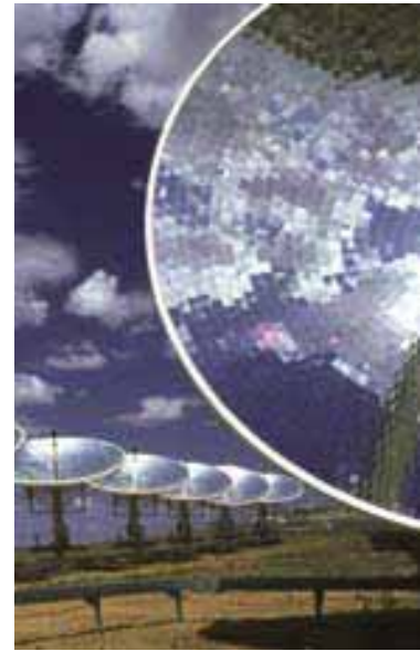
Solar power plant in Whitecliffs, Australia
